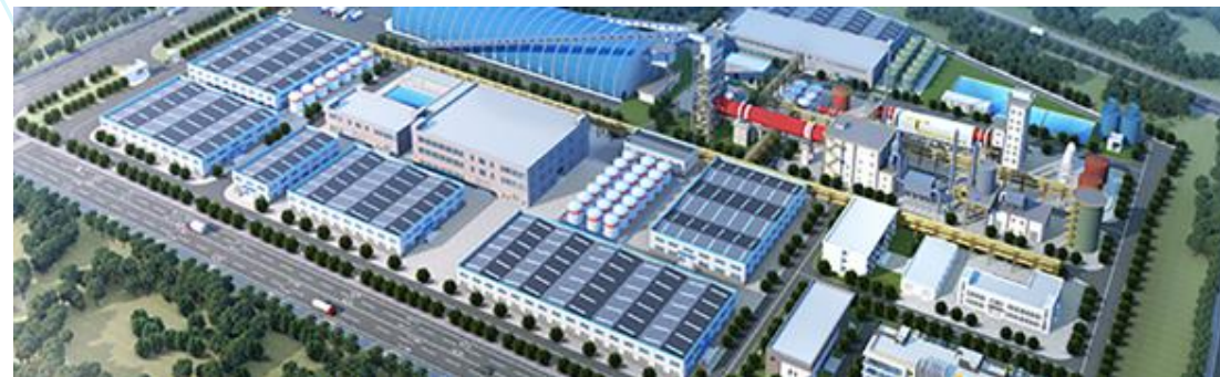
Hainan Mining's battery-grade Lithium Hydroxide Plant in Hainan Province
